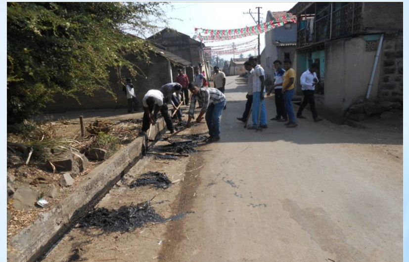
Drainage cleaning at Banewadi by NSS volunteer.
